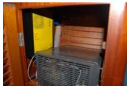
24v/220v Charger/inverter and 12v charger
